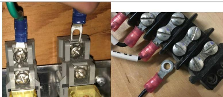
These connections are very secure but negate one of the advantages of using screw terminals, which is that the wire can be cut to size on-site.
