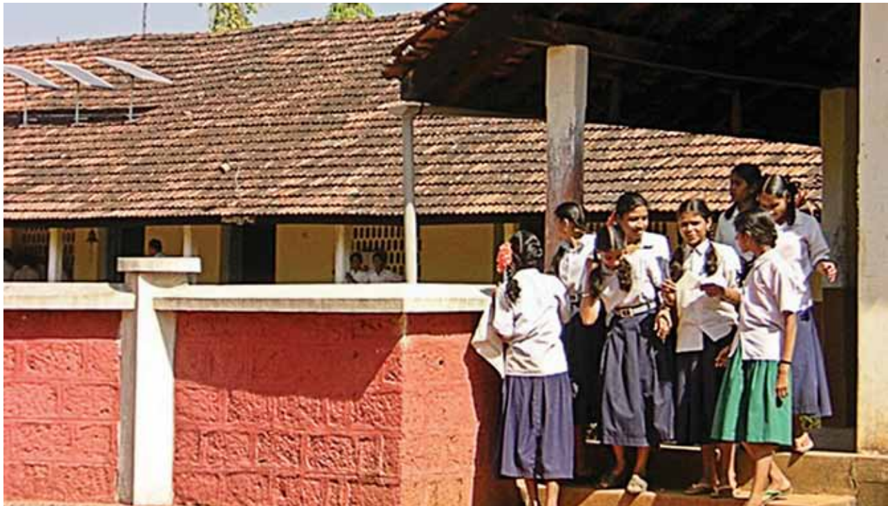
A school with an installed SHS in India
